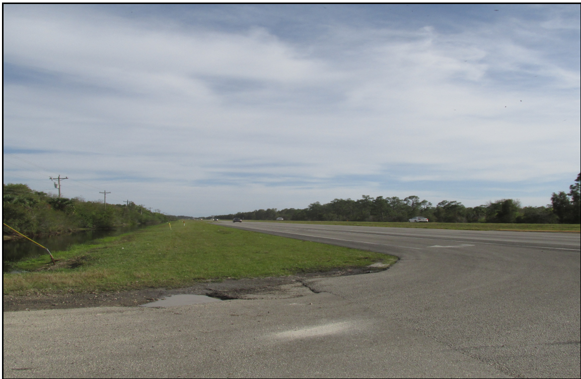
US HIGHWAY 41 FACING SOUTH
